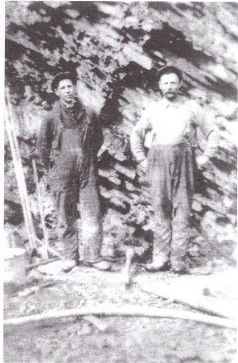
Trapps men working a shale bank for building carriage roads for the "new" mountain houses
